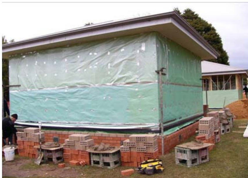
Figure 7: Taped and patched building wrap
