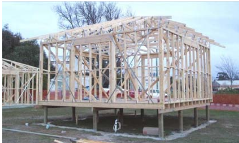
Figure 9: Test Cell 2 Wall and Roof Framing
