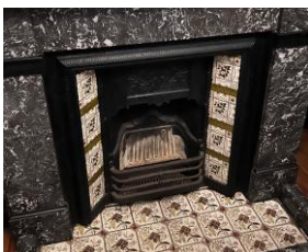
Figure 12.1 - Cast iron grate fireplace
