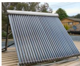
Figure 13.3 - Estimating solar system size – count the number evacuated tubes
