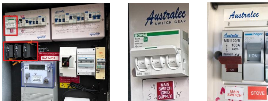
Figure 17.5 - Types of supply – Three phase = 3 mains switches, Single phase = 1 main switch
