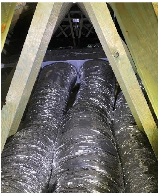
Distribution entirely outside the conditioned envelope
