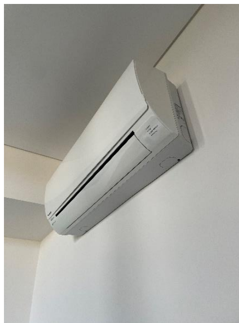
Distribution entirely within the conditioned envelope
