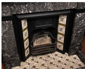
Figure 12.1 - Cast iron grate fireplace
