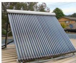
Figure 13.3 - Estimating solar system size – count the number evacuated tubes
