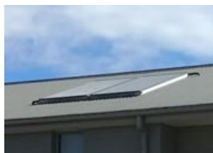
Figure 13.3 - Estimating solar system size – count the number evacuated tubes
