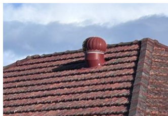
Figure 9.2 - Wind driven roof space ventilator
